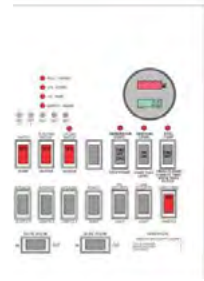
Command Center Panel
